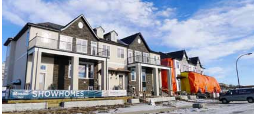
MOSAIC RIVERSTONE UNDER CONSTRUCTION IN CRANSTON.
