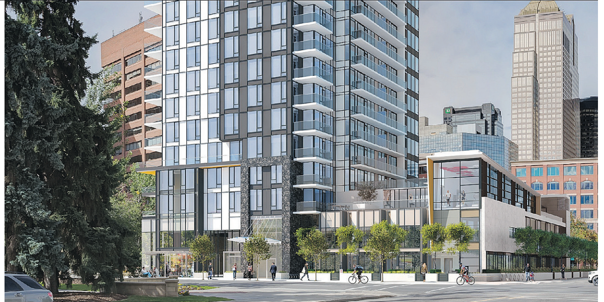
At 34 storeys, the Park Point condo tower will be the tallest building in the area. QUALEX-LANDMARK
