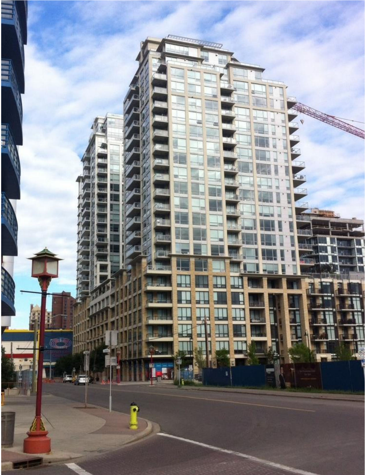
The Waterfront condo project is the largest condo project in Calgary's history.
