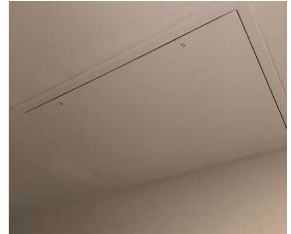
ENERGY RECOVERY VENTILATION ACCESS PANEL
