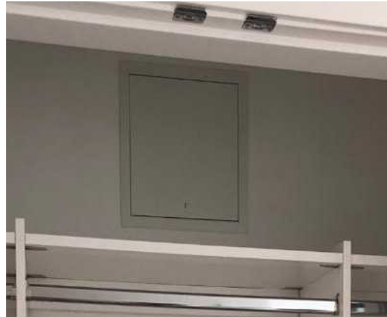
BATHROOM BASEBOARD HEATER ACCESS PANEL (THERMOSTAT 2 ONLY IN SOME SUITES)
