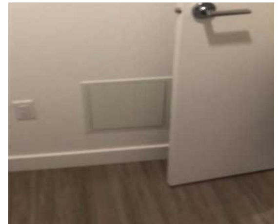
DOMESTIC WATER ACCESS PANEL
