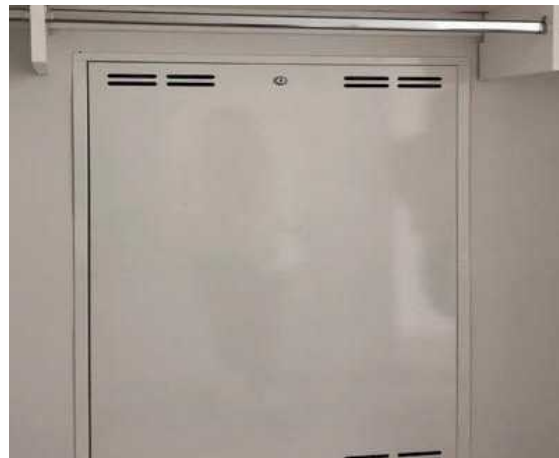
FAN COIL UNIT ACCESS PANEL (THERMOSTAT 1)
