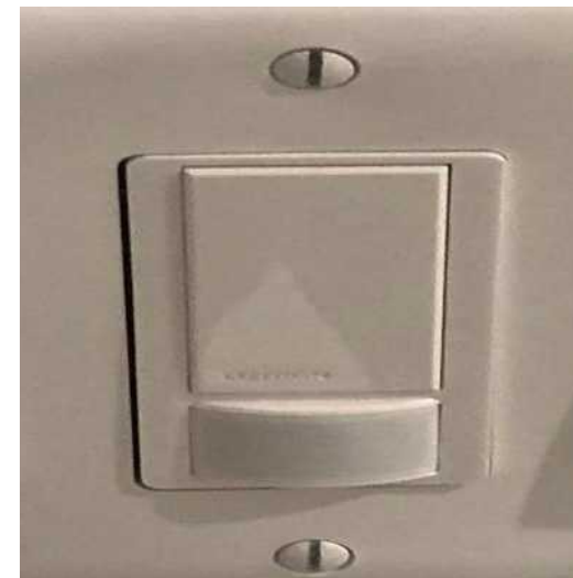
VENTILATION- 2ND BATHROOM
