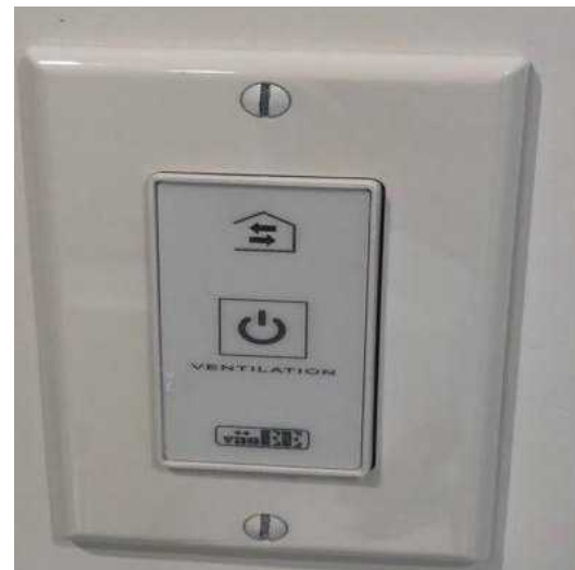
AIR VENTILATION MASTER BATHROOM
