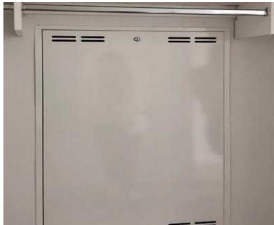
FAN COIL UNIT ACCESS PANEL (THERMOSTAT 1)
