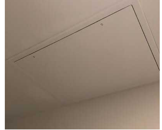
ENERGY RECOVERY VENTILATION ACCESS PANEL
